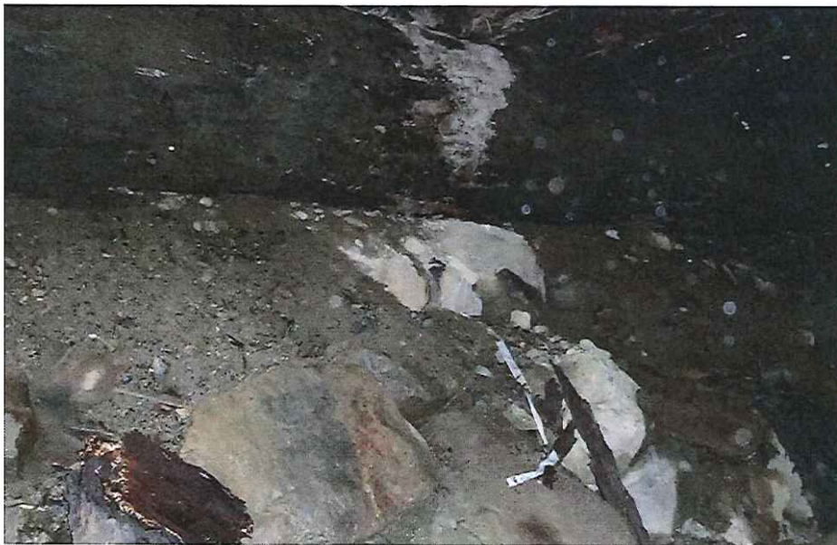
CK2236 Right Abutment
