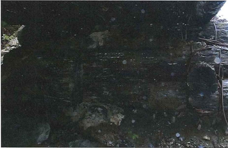
CK2236 Left Abutment
